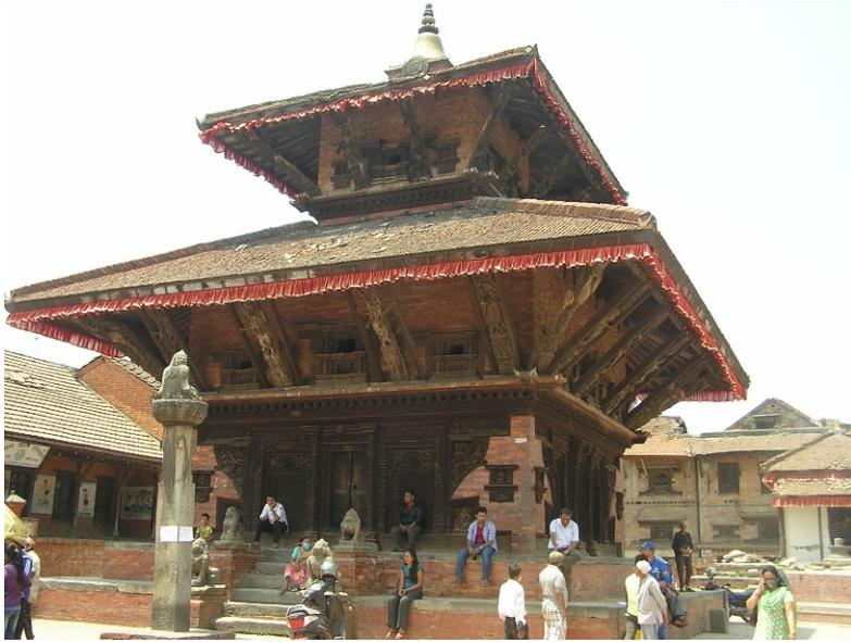
Most of the temples were built in pagoda style, having timber frames and brick masonry walls. The walls were of random rubble masonry core and dressed with brick masonry.
