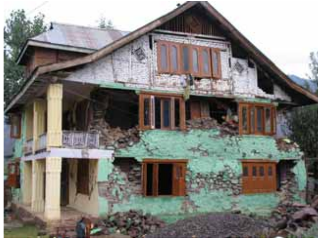
Figure 6. Timber-laced masonry in gable wall suffered little damage whereas extensive damage in stone masonry wall rendered the building unsafe at Uri.
