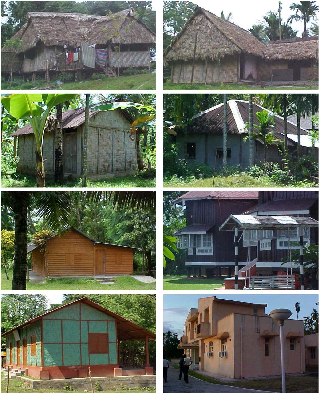
**Figure 9:** Transition of constructional strategies in Andaman & Nicobar Islands from traditional wooden construction with thatch roof to modern reinforced concrete frame buildings with sloped/flat RC slab roof.
