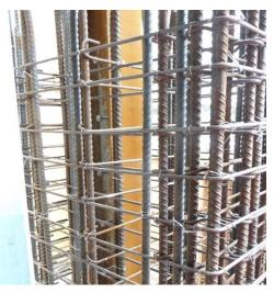
*Figure 3. Column reinforcement is visible before the concrete is cast. The reinforcement consists of vertical bars that resist bending, and horizontal ties that stop the column concrete from disintegrating and dislodging.*
