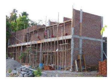
Figure 2. A confined masonry house under construction.
