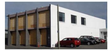
Figure 1. An earthquake damaged building. The strength and stiffness of the long white-colored masonry walls have prevented damaged. A more flexible structural system acting across the building has led to larger movement and damage to the front façade. It is temporarily covered with sheets of plywood.
