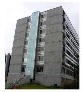
Figure 2. The seismic retrofit of this hospital building included two new structural walls and foundation at each end.
