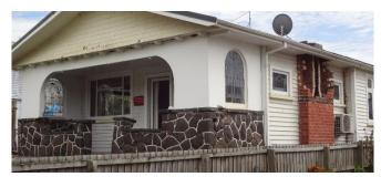
*Figure 3. A brick chimney has broken off at roof level and fallen. Most of the remaining chimney is damaged (N. Allaf).*
