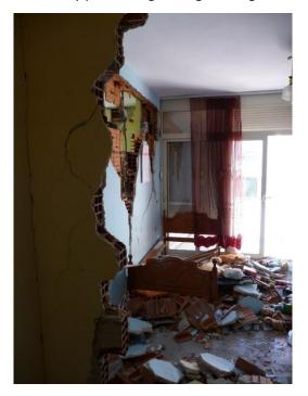
Figure 2. Walls damaged by earthquake shaking pose risk to life.
