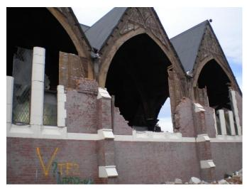
Figure 4. An earthquake has destroyed most of the brick cladding and glazing of this building.
