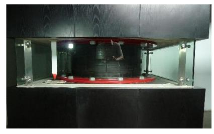
*Figure 4. A circular rubber bearing containing many thin steel plates is located between the bottom of every column and its foundation to isolate the building from horizontal earthquake shaking.*
