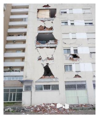
Figure 2. An example of an earthquake damaged building where the infill walls have not been carefully designed to allow for forces and movements during an earthquake.
