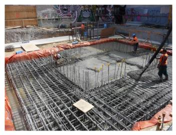
*Figure 3. The foundations of a building under construction. Engineers have followed codes to determine the amount of reinforcing steel and its correct location.*
