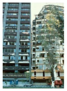
Figure 2. Two buildings have pounded each other with one far more seriously damaged than the other.
