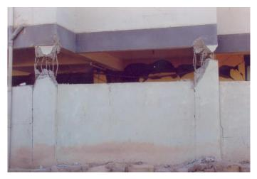
Figure 4. Earthquake-damaged short columns.
