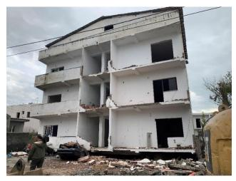
Figure 4. This soft story building lost its ground floor during a moderate earthquake (N. Vesho).
