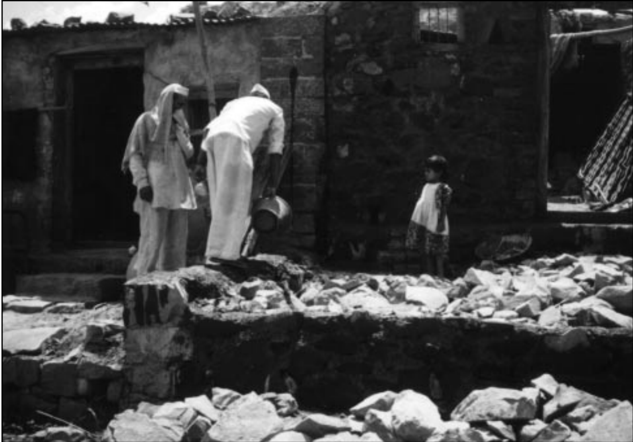
Figure 46 Beneficiaries participated in the construction in the repair and strengthening villages. Here they are curing masonry by hand-pouring water from containers.
