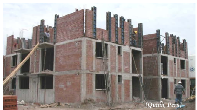
Fig. 5. A building in construction using confined masonry [Quinn, Peru]
