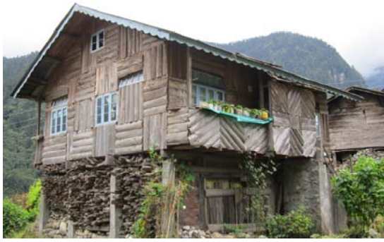
Fig. 3 Traditional Shee-khim house which suffered negligible damage
