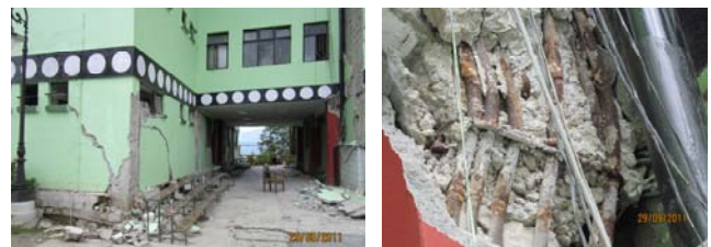
Fig. 2 Damages observed in state secretariat building
