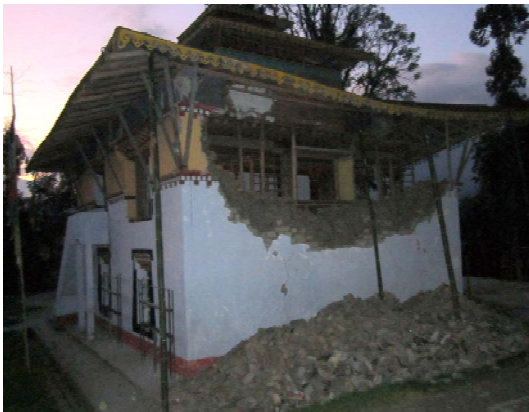
Fig. 4 Partial collapse of stone masonry walls of a monastery temple at Mangan
