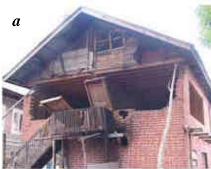
Figure 7. Failure of supporting walls for the roof in a traditional building using Taq system of masonry at Baramulla.
