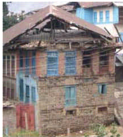
Figure 7. Failure of supporting walls for the roof in a traditional building using Taq system of masonry at Baramulla.
